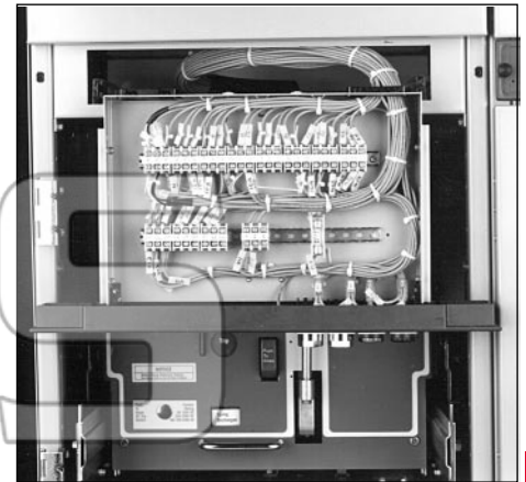
Breaker Cell Terminal Block Tray Withdrawn and in Inspection Position
