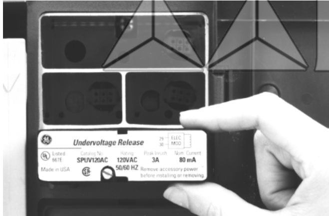
Figure 3. Inserting the Undervoltage Release into the accessory compartment.
