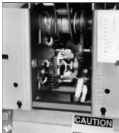
Figure 9: Spring charging motor
