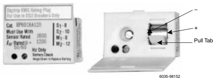
Figure 30: Rating Plugs Shown with Covers Closed and Open
